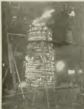
Typical Foundry Scene. This shows how castings are poured on end with larger risers so as to produce a dense homogenous metal in the casting.
